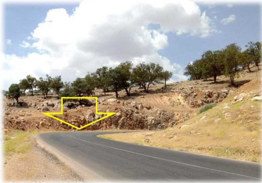
Trench excavation site
